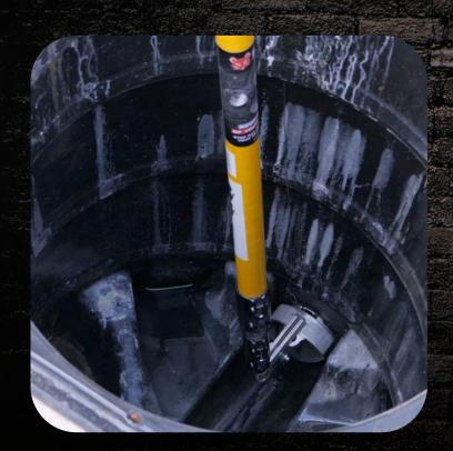
To make installation even simpler, and to allow fitters to access tight drains, we also developed the RatGate Installation Pole.
